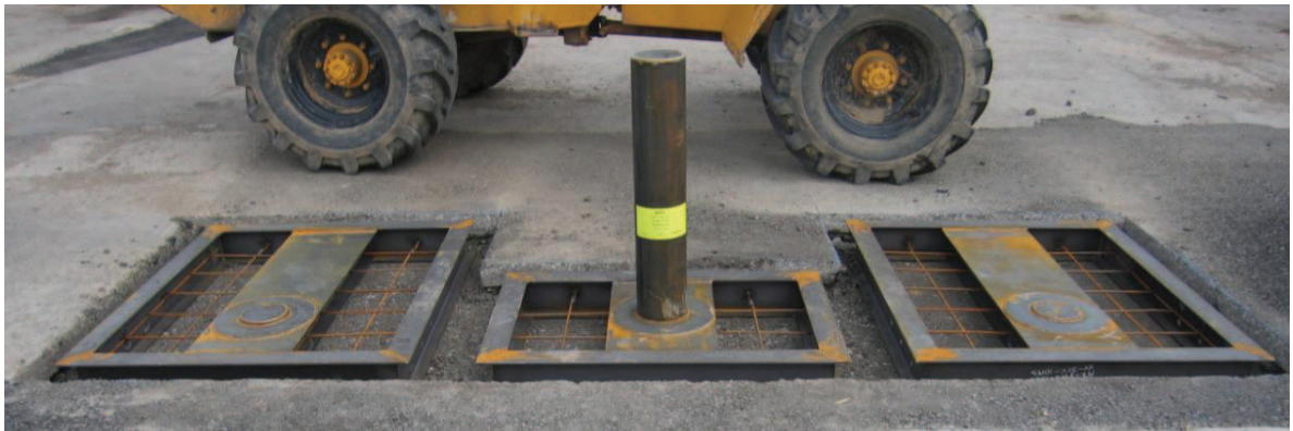
Figure 1 – Shallow Mount Units in Position
