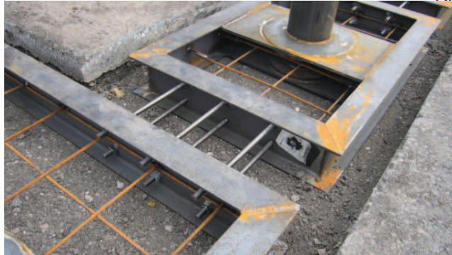
Figure 2 – Connecting Bars fastening Foundation Units
